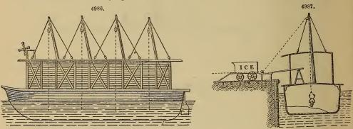
standard, kept upright by stays and furnished with a pulley. The ice is lifted by a lazy tongs attached to the hauling rope, which is so arranged as to swing it immediately into the ice cart, Fig. 4987.
